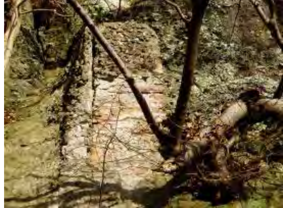
Figure 432 Brick chimney under artificial stone
