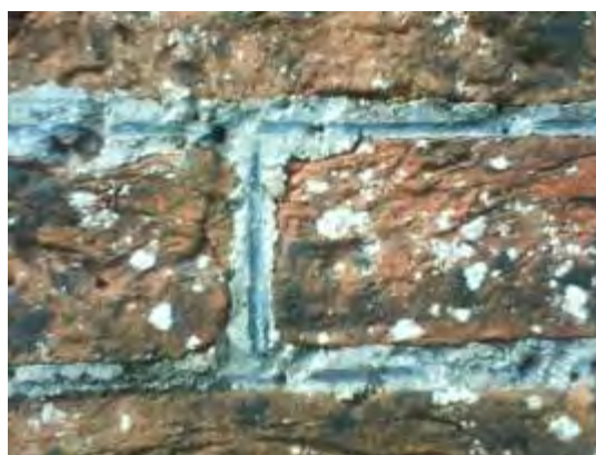
Figure 404 Lime pointing in walled garden wall 2009
