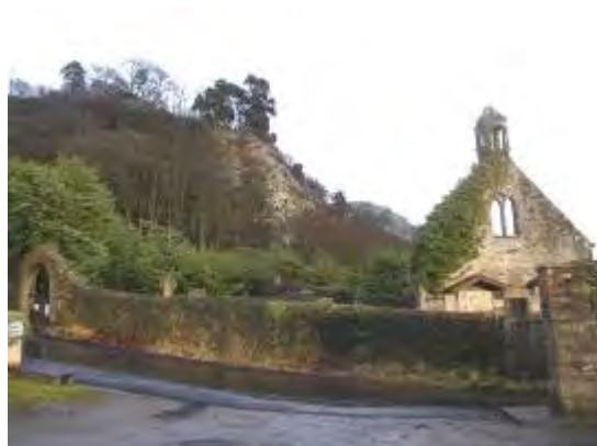
Figure 408 View to east from in front of Garden Cottage 2009
