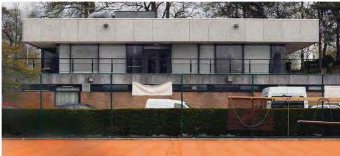
Figure 217 East elevation of Gannochy Trust Pavilion. Note the closed blinds on the upper level, the car parking and the fenced off tennis courts in front.
