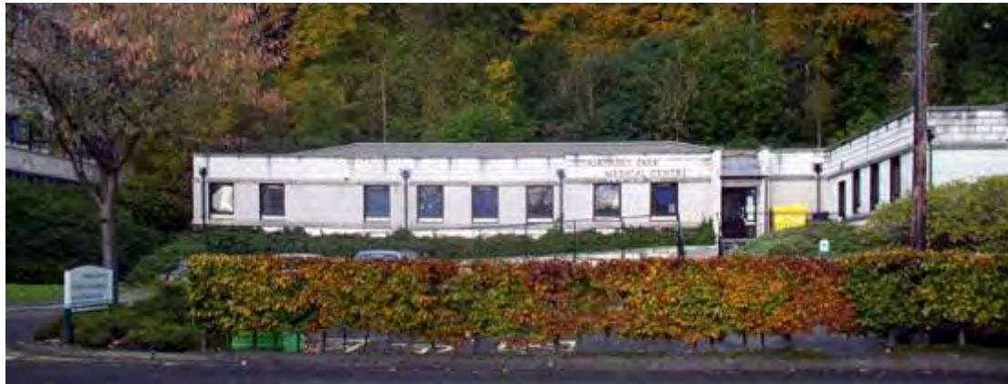
Figure 202 Airthrey Park Medical Centre 2008
