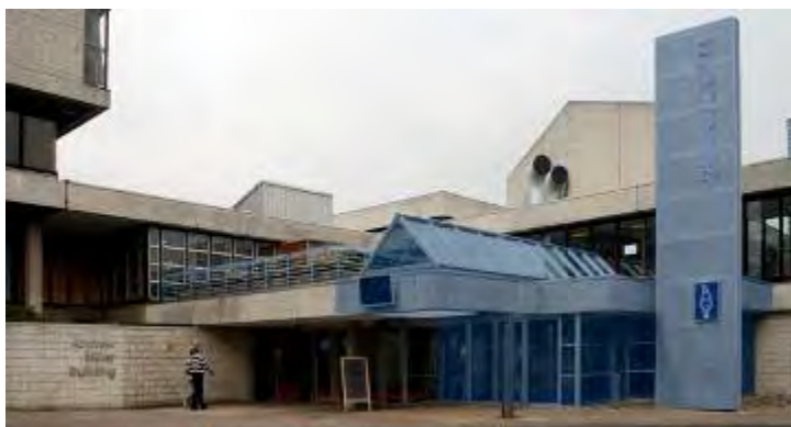
Figure 161 Architectural ‘clutter’ created with the refurbishment of the MacRobert Centre highlighted in blue.
