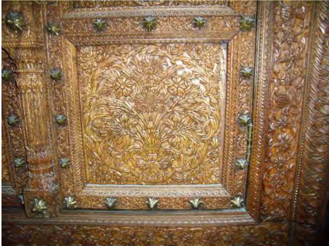
Figure 364 Detail of panelling on Indian doorway
