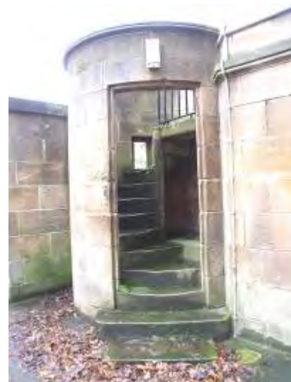
Figure 355 Stair to conservatory 2009
