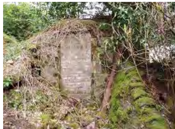
Figure 248 Icehouse, blocked door 2009
