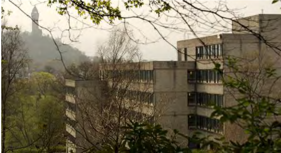
Figure 195 East elevation of A.K. Davidson Hall, looking towards the Wallace Monument.
