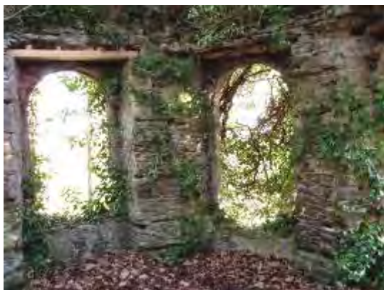
Figure 443 Windows to south east and south 2008
