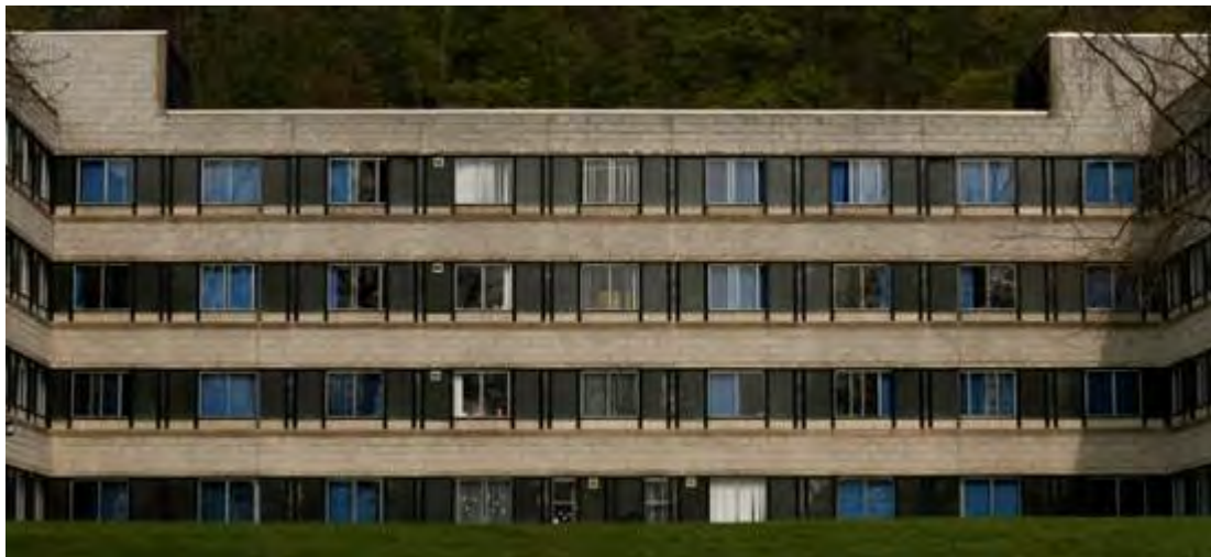
Figure 198 General view of Muirhead House, with the original fenestration.
