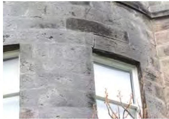
Figure 351 Slipped keystone first floor 2009
