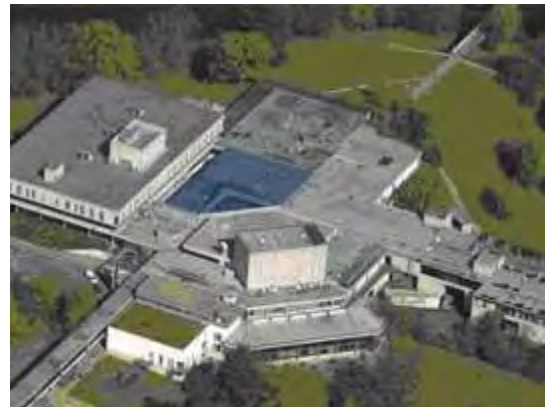
Figure 172 2007 Oblique aerial view from south-east with covered atrium highlighted in blue. RCAHMS edited by S&B
