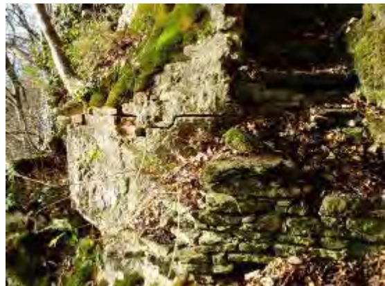
Figure 436 Lower portion of steps to platform 2008
