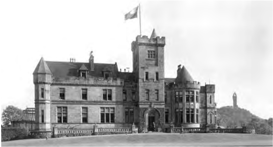
Figure 327 North front 1937 StAU
