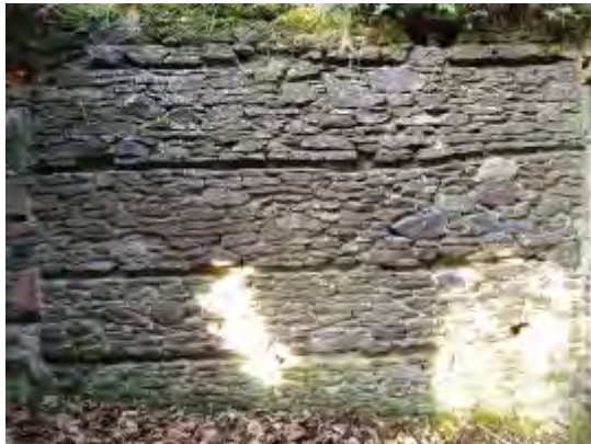
Figure 441 North wall, interior
