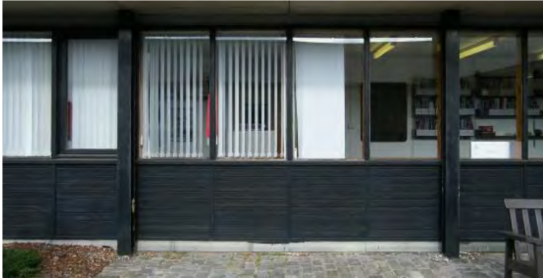
Figure 122 The same area as in Figure 51 above as viewed from the sculpture courtyard, showing the windows with vertical mullions.
