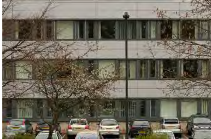
Figure 141 South elevation of Cottrell showing the replacement cladding and fenestration
