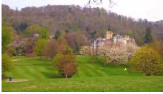
Figure 377 View of castle from south west, concealed behind small trees 2009
