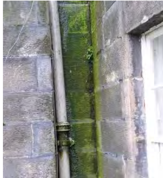
Figure 352 Leaking pipe 2009
