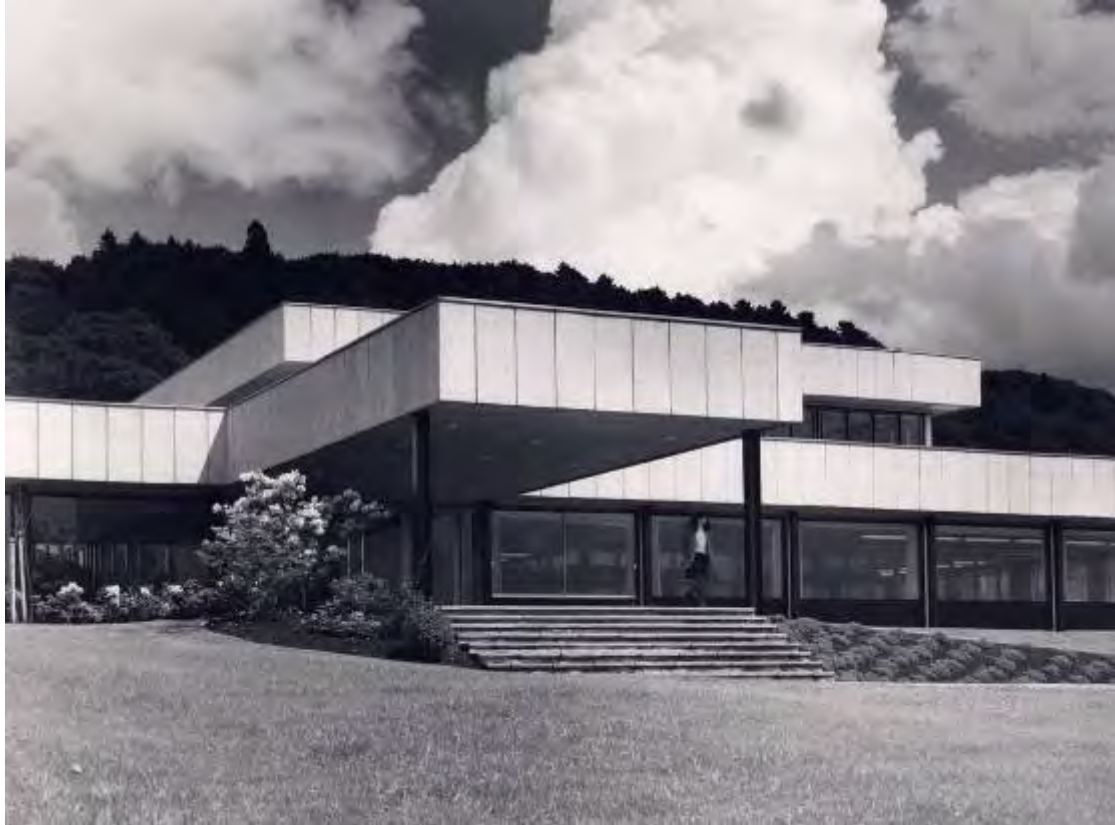
Figure 119 Pathfoot entrance canopy, projecting from the building as intended UoSA
