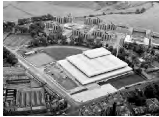
Figure 108 Aerial view of the Royal Commonwealth Pool, 1969. Scran/Scotsman Publications
