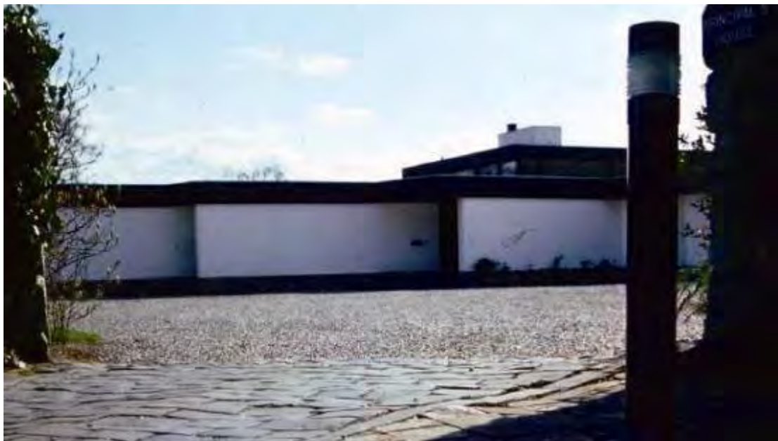
Figure 252 Undated 1960s-70s photograph of Principal's House with original entrance and white rendered water tank and chimney Robert Steedman
