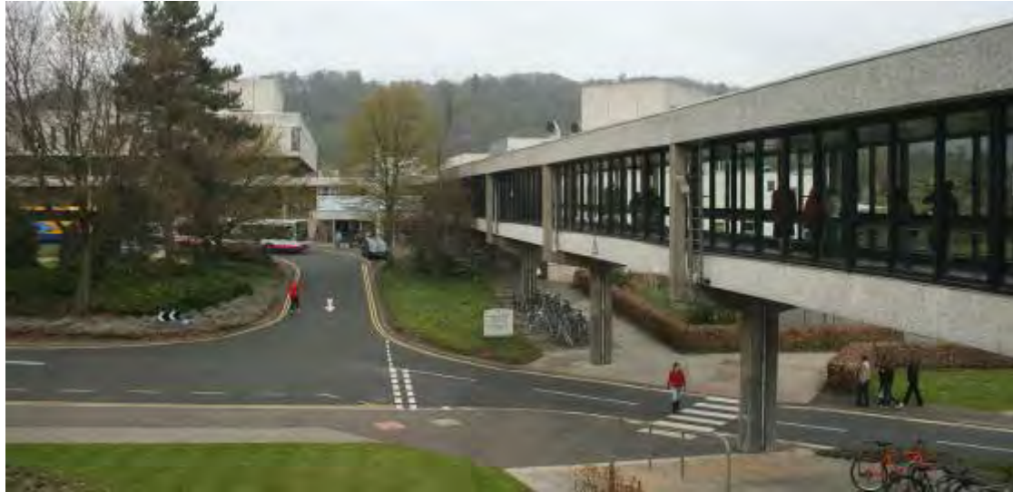
Figure 166 External view of the link bridge
