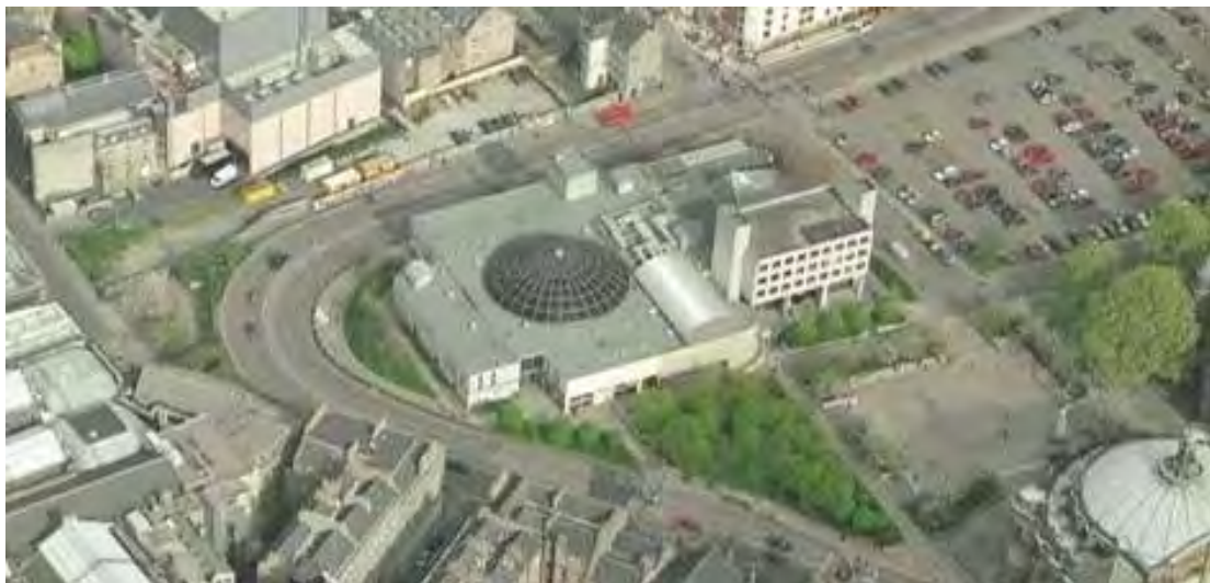
Figure 21 Oblique aerial view of the Students' Amenity Centre with the large dome covering the atrium space on the interior. RCAHMS
