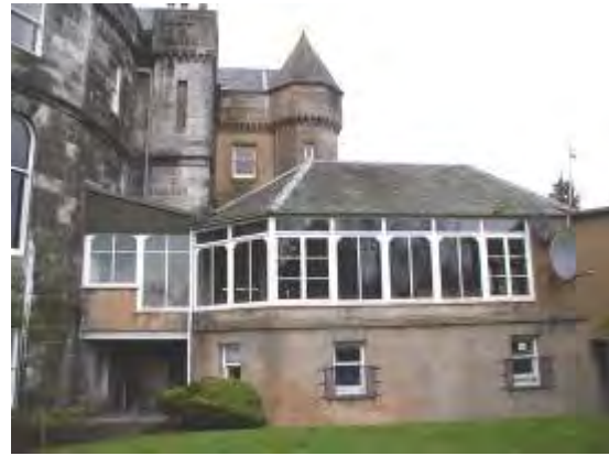
Figure 353 South elevation of conservatory 2009
