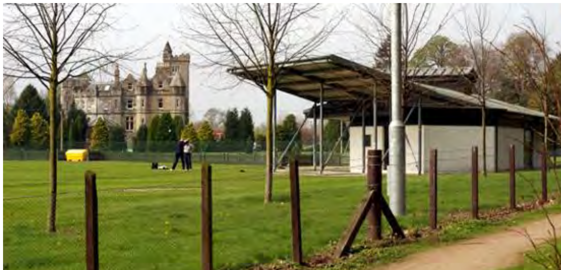
Figure 349 Sports Pavilion with Airthrey Castle in the background 2009
