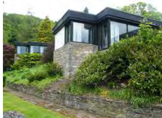
Figure 244 Re-used stone forming bases for Nuffield Houses 2009
