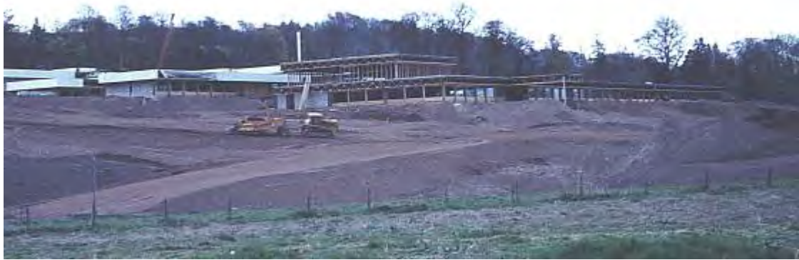
Figure 113 Pathfoot under construction, c1968. UoSA
