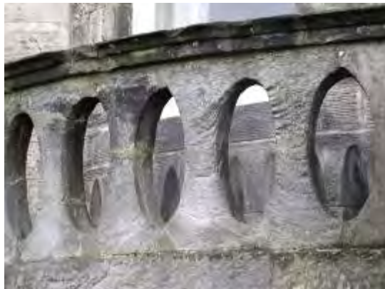
Figure 350 Detail of balustrade 2009
