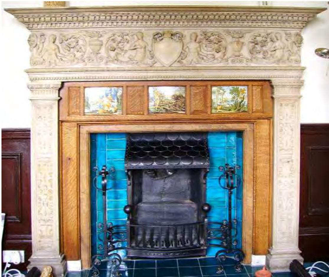
Figure 337 Former Dining Room, Italian Renaissance carved limestone chimneypiece, with inset pictorial Majolica tiles, and late 19 th century oak setting and wrought iron chimney grate
