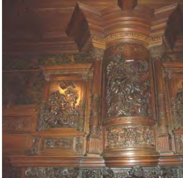
Figure 336 Detail of panelling around fireplace, hall. Includes Flemish and Italian carving of early-mid 17 th century
