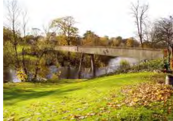
Figure 205 Footbridge from east 2008
