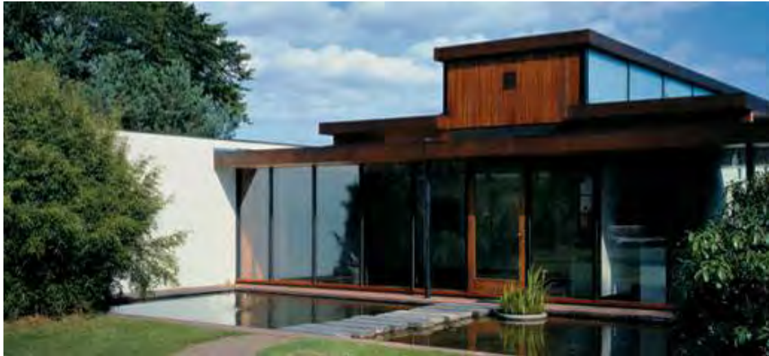
Figure 104 Exterior of the Louisiana Museum of Modern Art, showing similar arrangement of glazing, roof structure, and clerestory as found at Pathfoot. www.louisiana.dk
