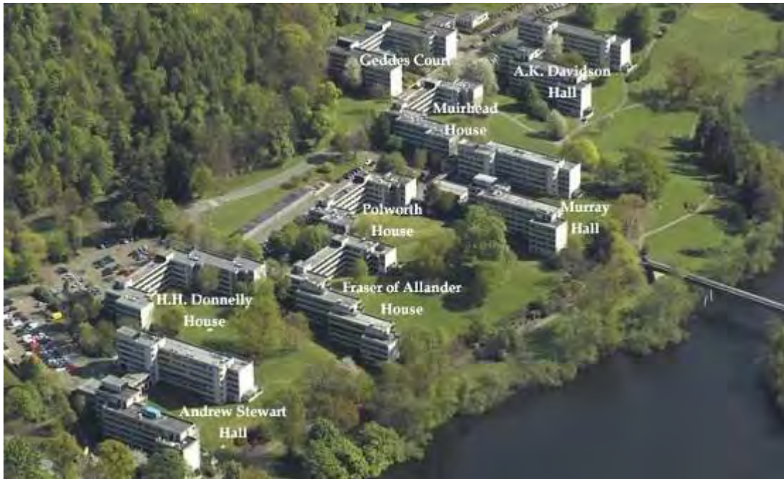
Figure 193 Oblique aerial view from 2007 of the Students' Residences, annotated with the building names. RCAHMS edited by S&B
