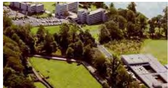
Figure 98 Detail of aerial photograph showing planting of trees to east of Pathfoot 1976 British Geological Survey
