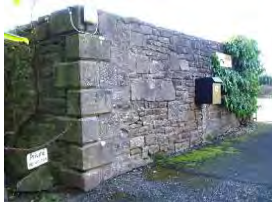
Figure 234 Quoins on former wall of steading
