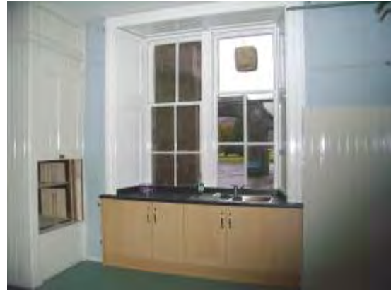
Figure 365 19 th century boarding and service lift in former kitchen 2009
