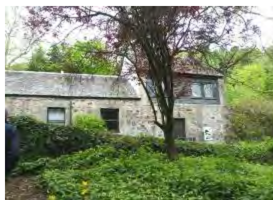
Figure 285 Airthrey Cottage, east block 2009
