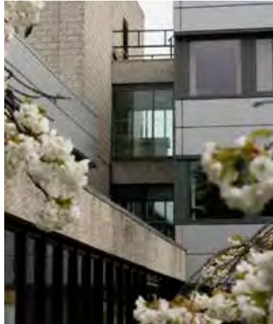
Figure 140 Original and replacement cladding and fenestration
