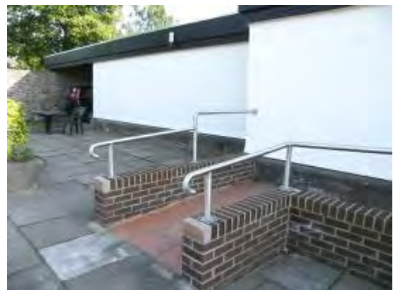
Figure 273 Ramp and steps 2008
