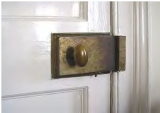
Figure 308 18 th century door and lock, Room 36
