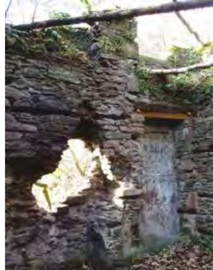
Figure 446 West wall with recess and remains of fireplace and chimney
