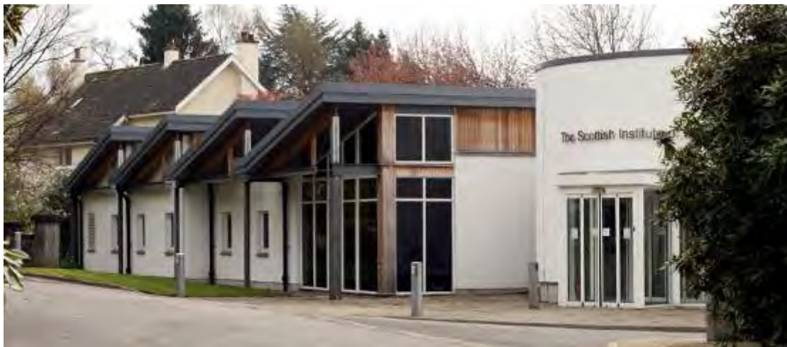
Figure 471 Main entrance to Scottish Institute of Sport within extension to villa
