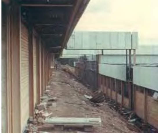
Figure 115 Pathfoot under construction, showing area between different terrace levels. UoS
