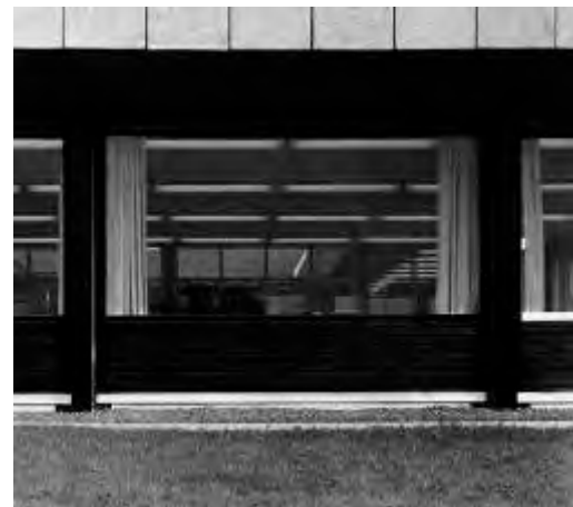
Figure 114 A typical prefabricated panel with full-width window. UoSA
