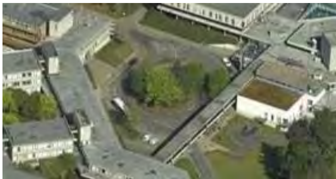
Figure 168 Oblique aerial view of Queen's Court. RCAHMS
