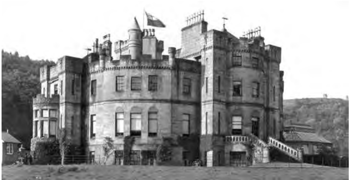
Figure 328 View from south west 1937 StAU
