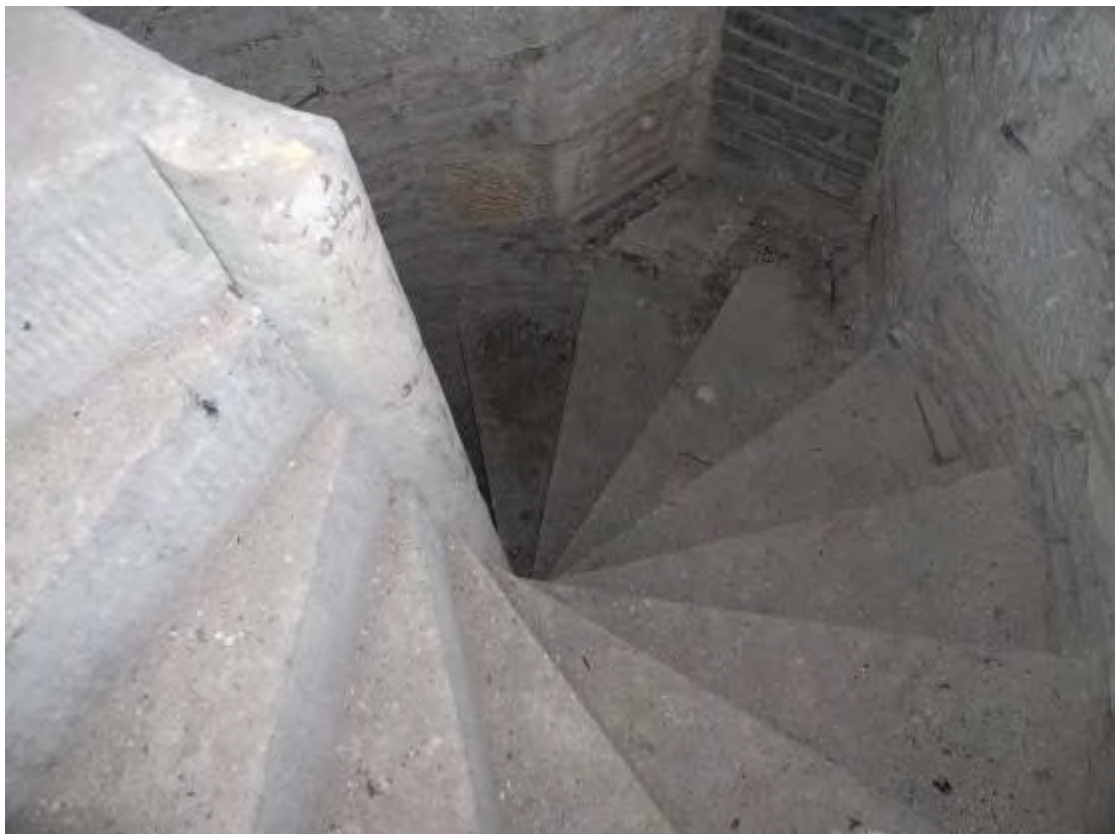
Figure 375 Spiral staircase in East Lodge 2009
