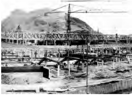
Figure 107 Royal Commonwealth Pool under construction in 1968. Scran/Scotsman Publications
