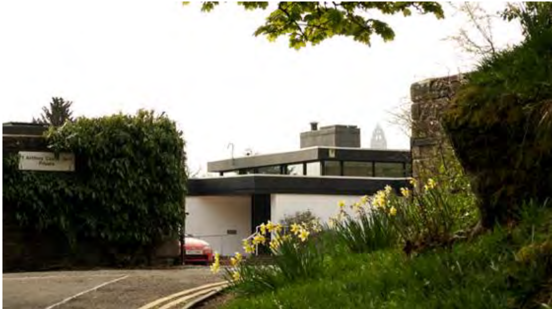
Figure 253 Restricted view of the Principal's House from the access drive, ensuring privacy, but also adding drama on arrival into the generous courtyard, with the Wallace Monument in the distance providing a hint of the views provided within. 2009
