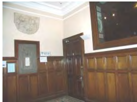
Figure 357 Panelling and inset carved reliefs in Lobby, with opening to Hall
