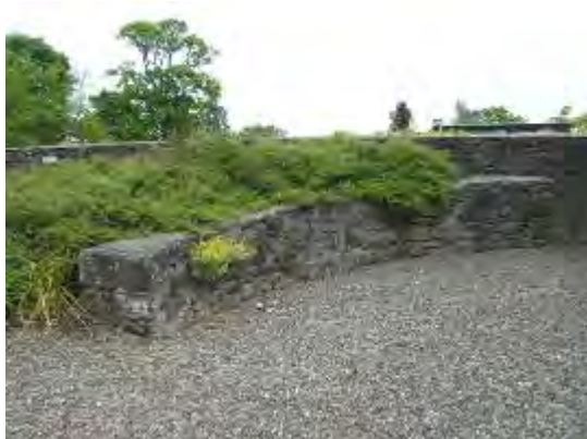
Figure 243 Curved wall of former horse gin, with walls of former farm building and roof of Principal's House beyond 2009
