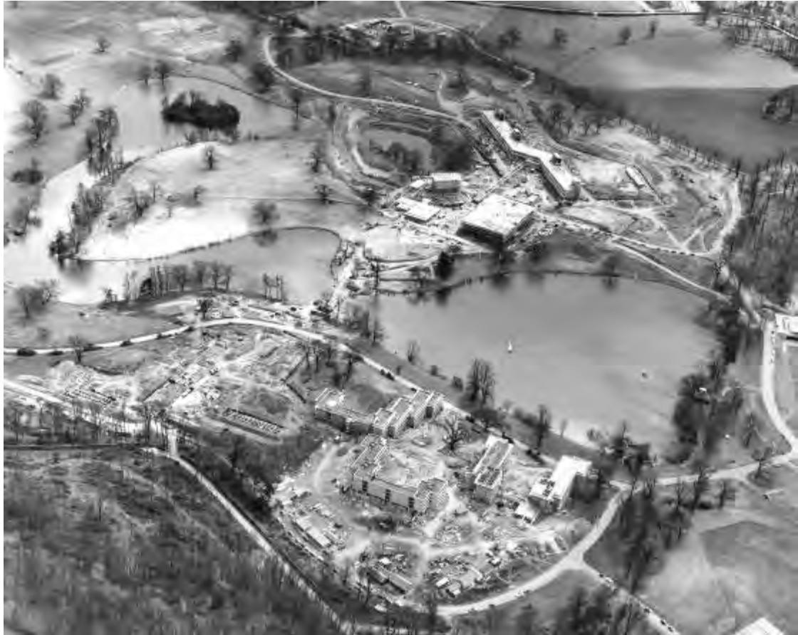
Figure 192 Aerial photograph showing construction of students' residences UoSA
