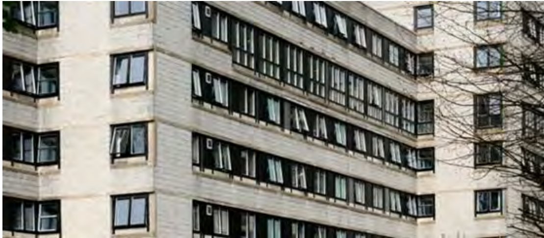
Figure 200 General view of replacement fenestration – note the bold black frames and the top-hung hinged opening.
