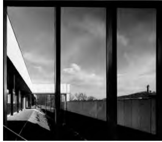
Figure 116 View over roof of lower terrace from stair between levels. UoS
