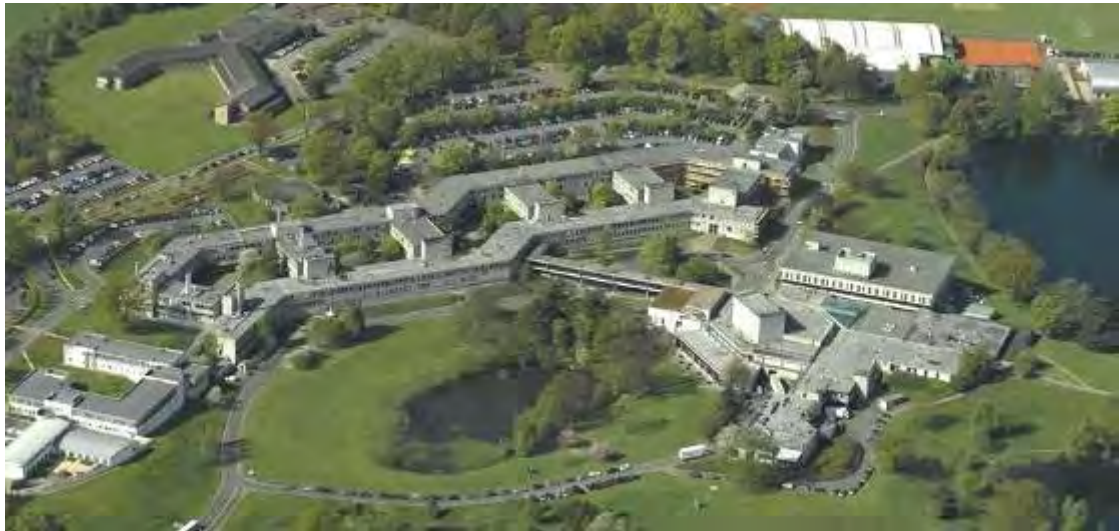
Figure 131 Oblique aerial view from 2007 showing the central area buildings. RCAHMS
