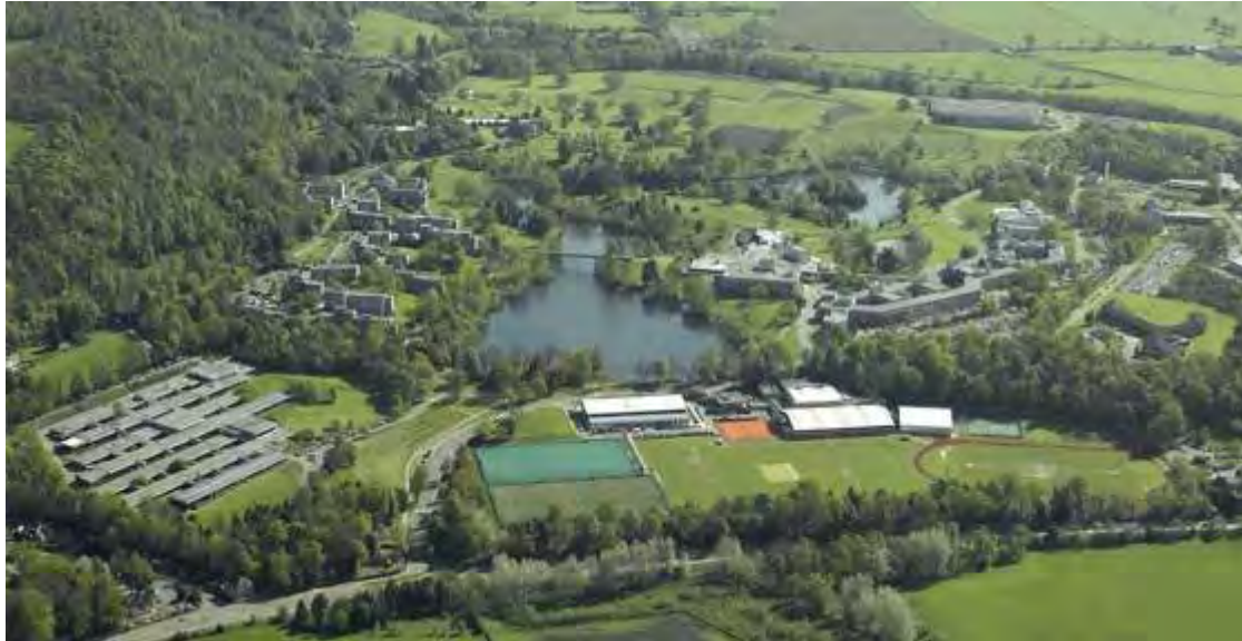
Figure 101 Aerial photograph of campus, Pathfoot to left 2007 RCAHMS
