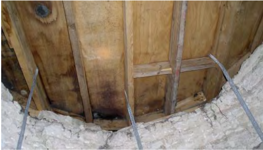
Figure 374 Staining on ceiling of East Lodge 2009
