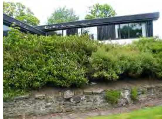
Figure 274 Flaking paint on fascia 2009
