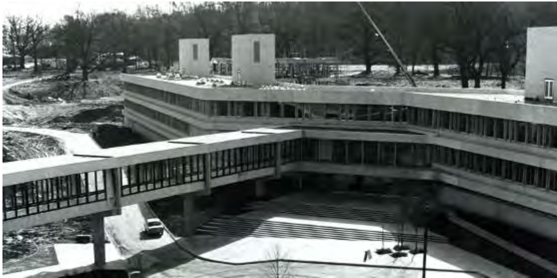
Figure 134 The north elevation of the first phase of the Cottrell Building nearing completion c1970. Note the start of construction of one of the 'rib' blocks in the background. UoSA
