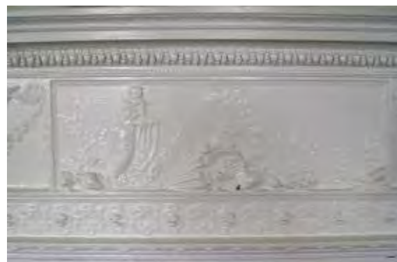
Figure 315 Detail of chimneypiece, Room 36
