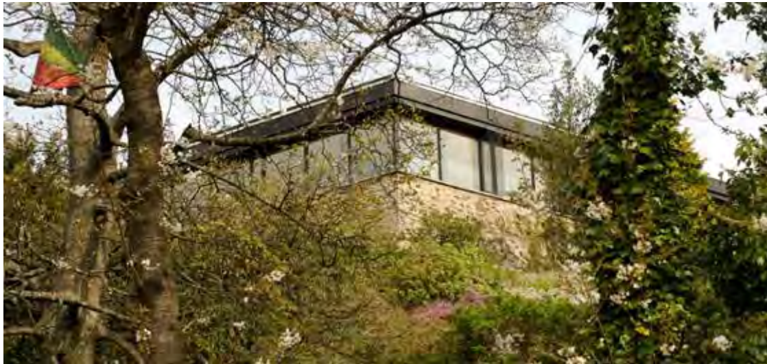
Figure 256 View of the Principal's House from road level showing the both the dramatic nature of the hill-top site and the integration with the surrounding landscaping 2009
