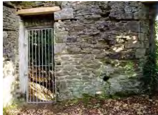
Figure 442 East wall, interior
