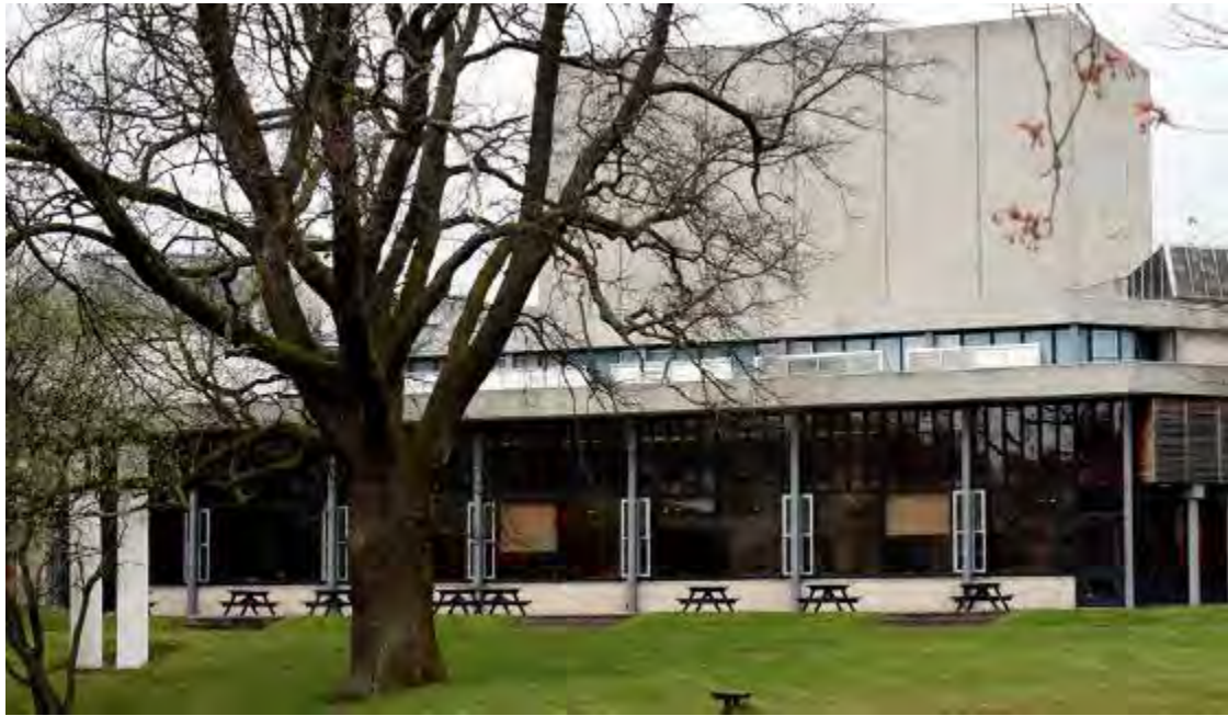
Figure 150 MacRobert Arts Centre with double-height dining space at the lower level and fly-tower behind.
