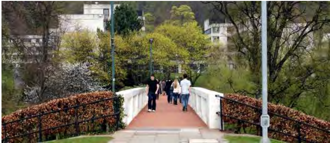
Figure 163 View of the footbridge looking towards the students' residences.
