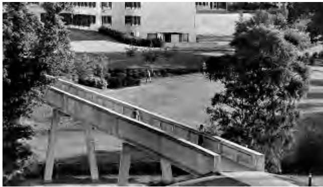
Figure 164 View showing the simplicity of the structure of the footbridge. UoSA
