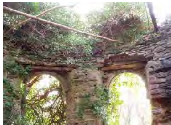
Figure 444 Windows to south and south west with crenellations
