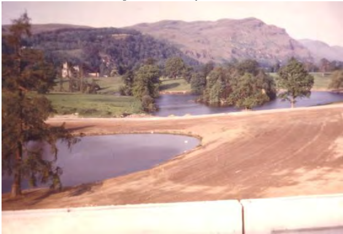
Figure 130 Construction of new road, dividing pond from loch c1968 UoSA
