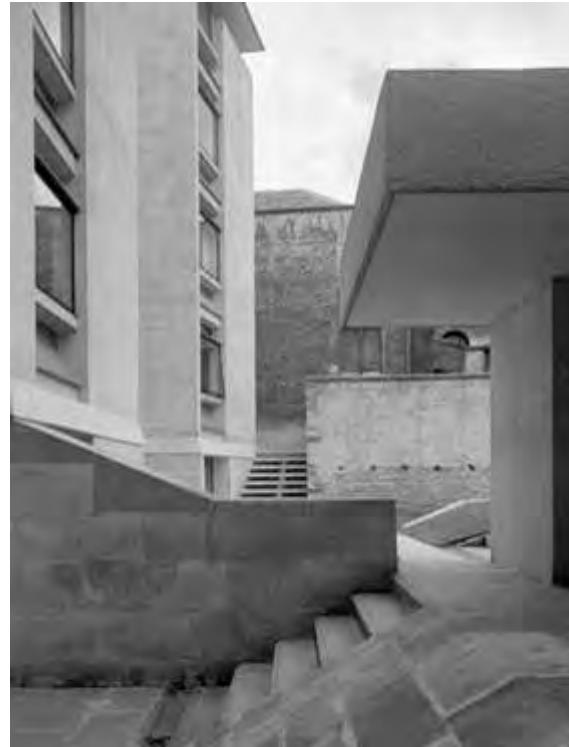
Figure 45 Powell and Moya accommodation blocks built at Brasenose College, Oxford. English Heritage NMR
